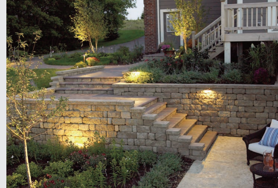
Above: Bayfield retaining wall in custom color.
